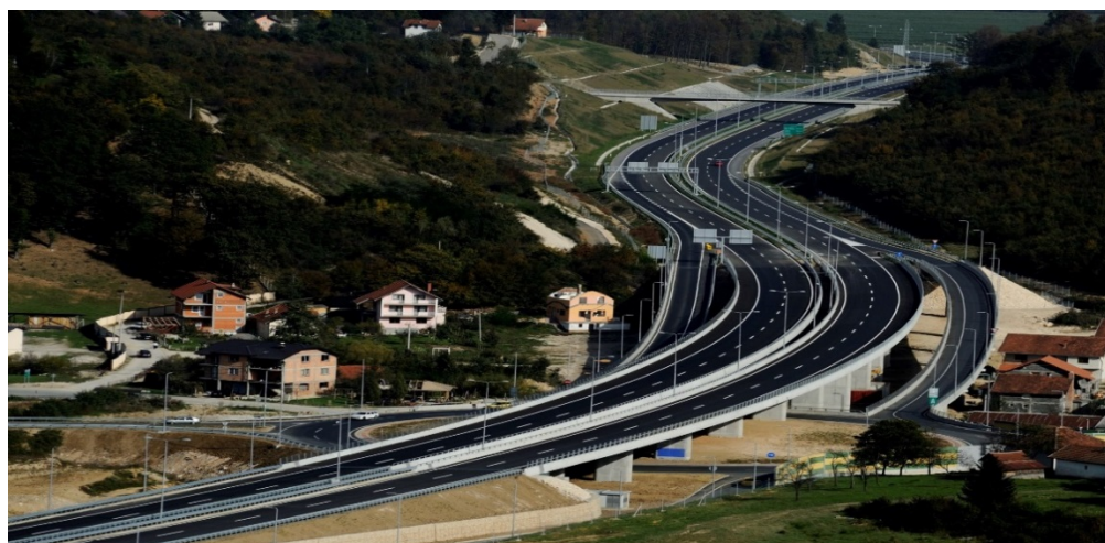
Newly built motorway on the Tarčin – Sarajevo – Zenica section on the Mediterranean Corridor in Bosnia and Herzegovina.
