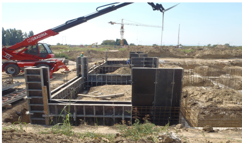
Construction of Pančevo Prison.
