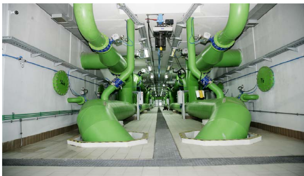
Existing water treatment facilities in Makiš 2 Water Treatment Plant.
