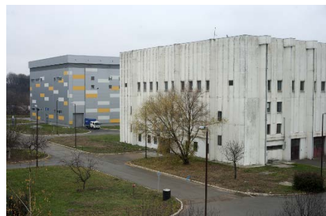
New and to-be-refurbished water treatment facilities in Makiš.
