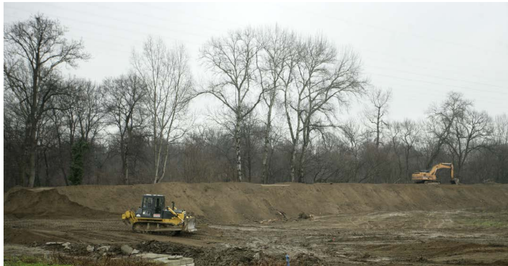
Preparatory works for future investments. December 2017.
