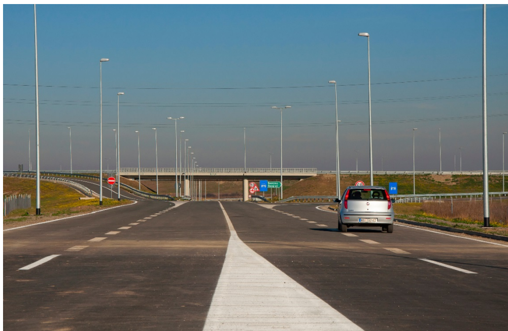
Existing infrastructure on the Orient/East-Med (CX) corridor in Serbia.
