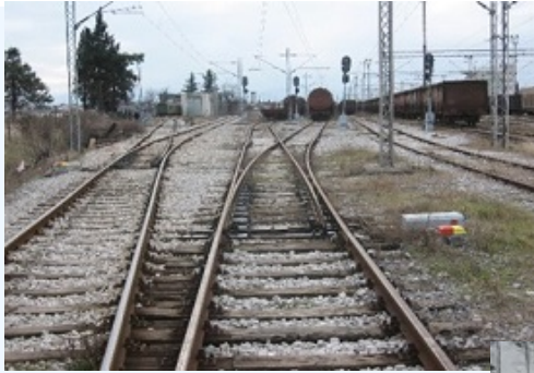
Podgorica Railway Station rehabilitation of signalization
