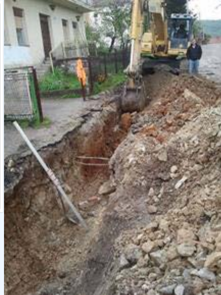
Sewerage network construction in Bosanski Petrovac
