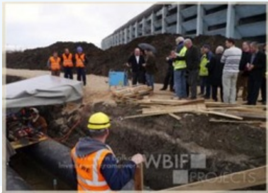
Donors visiting Pristina District Heating project works
