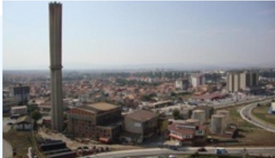
TERMOKOS Heating Plant in Prishtina
