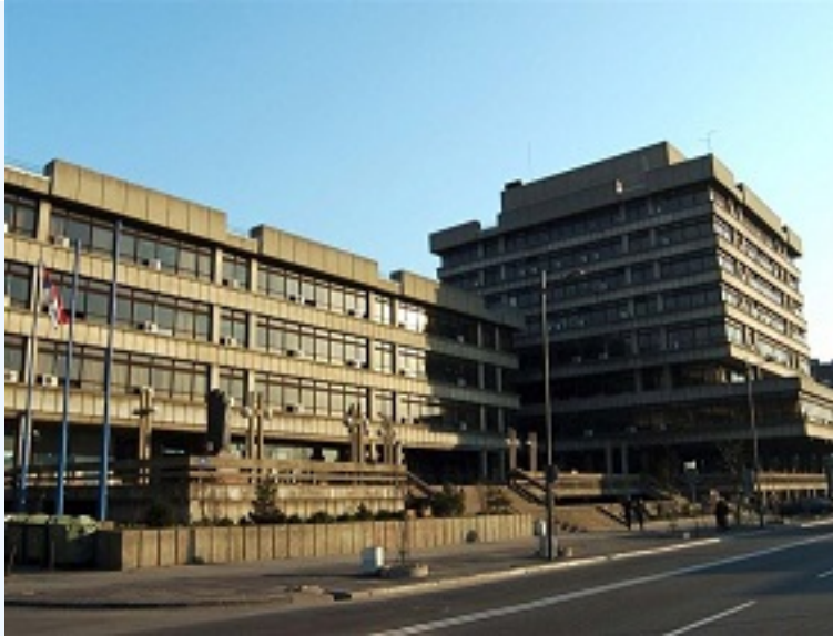
Palace of Justice (Building B)
