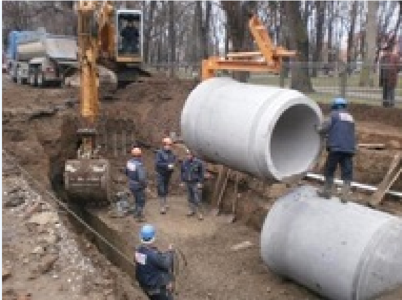
Bijeljina: Construction of collector No. 8
