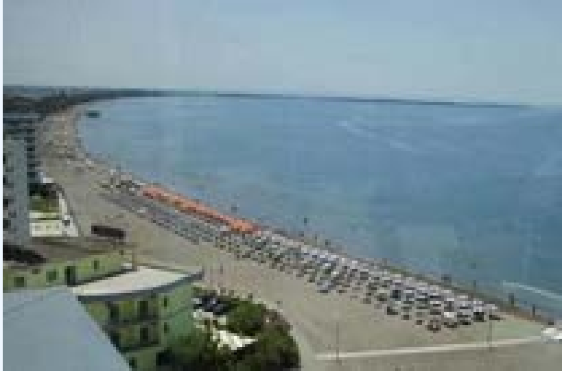
Shengjin beach where the sewerage network is implemented
