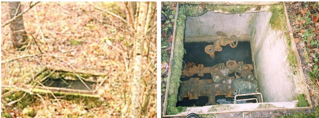
**Figure 8.22:** Inspection shafts on the route of the pipeline for the transport of kerosene to the airport Željava (Archive photo from 2003)
