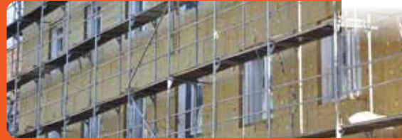
Flagship 6 • Renovation wave
