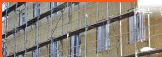
Flagship 6 • Renovation wave
