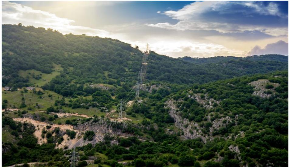
Trans-Balkan Electricity Corridor: Grid Section in Montenegro. The WBIF has provided €27.5 million in EU grants, including a €25.5 million investment grant under the Connectivity Agenda in 2015 for the construction of approximately 165 km long 400 kV transmission line and substations in Lastva and Pljevlja.
